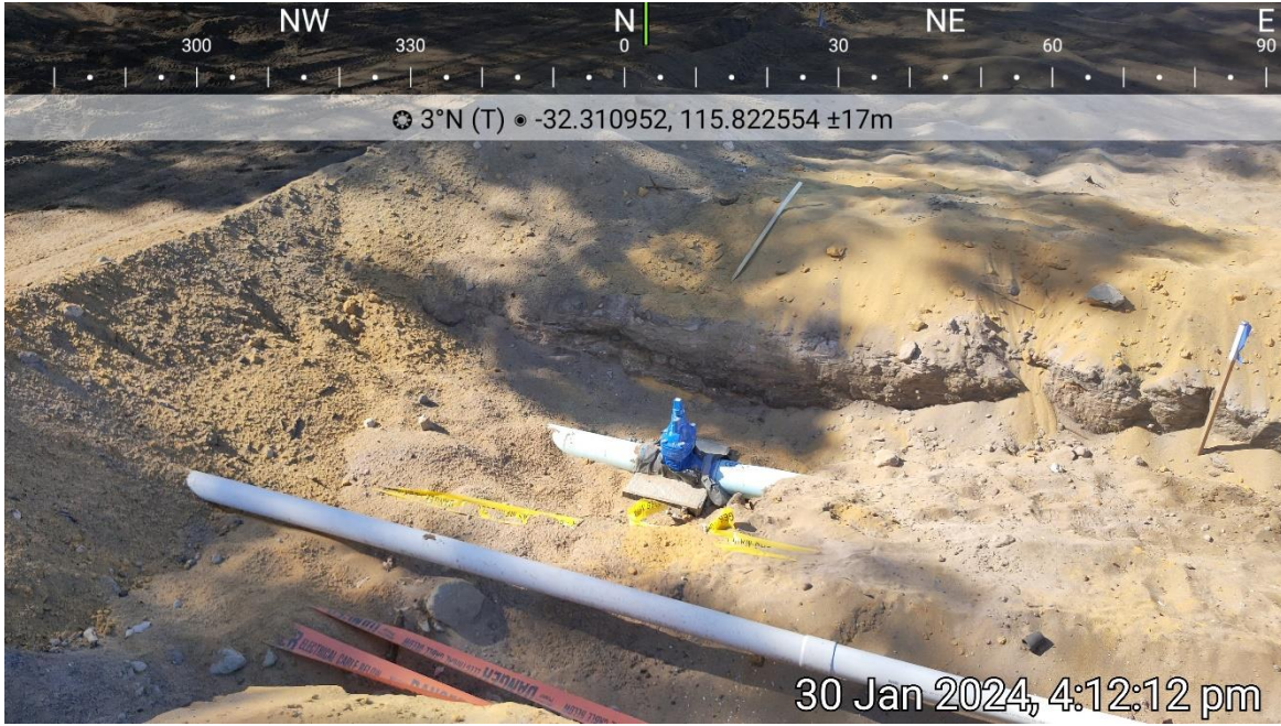
Plate 9: Evidence installation of hydrants and internal water reticulation is underway
