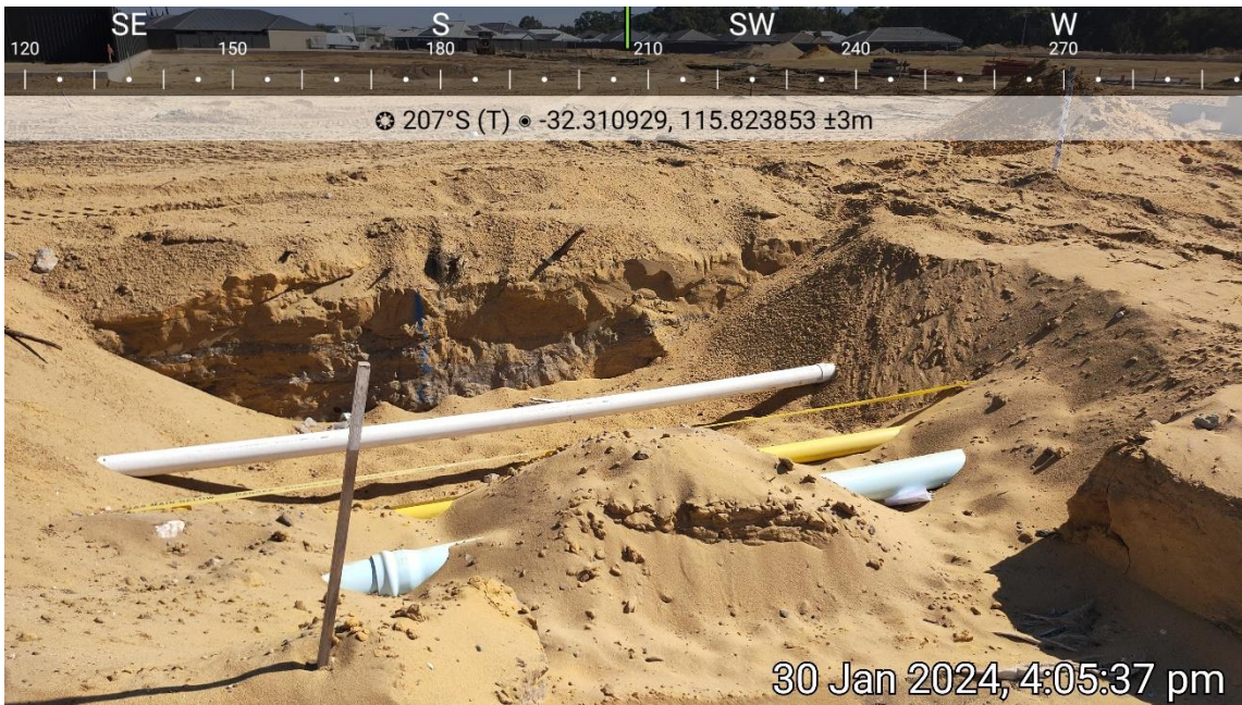
Plate 8: Evidence of installation of internal water reticulation is underway.
