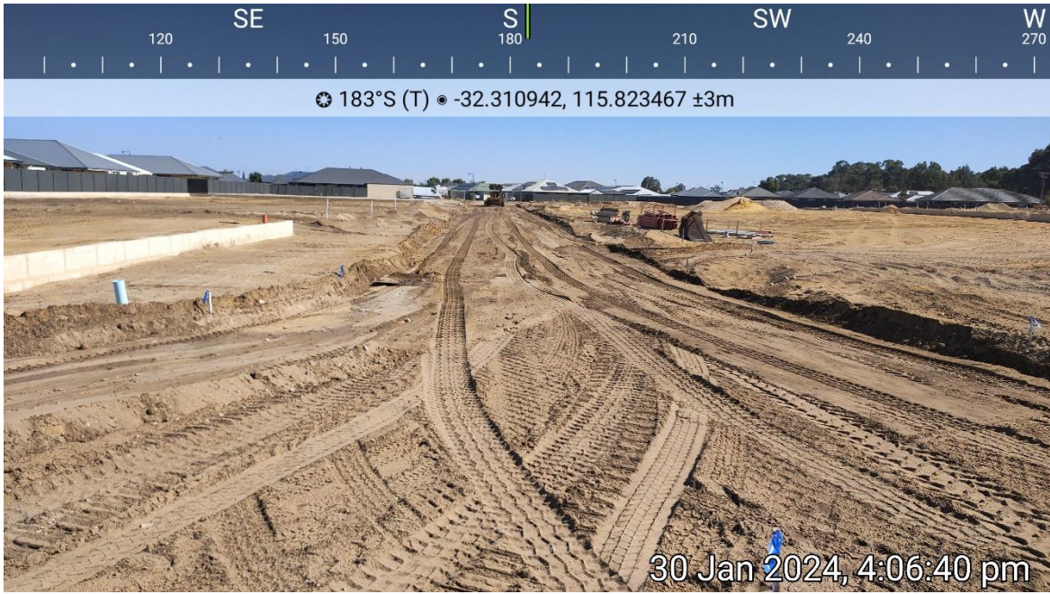
Plate 5: Evidence of construction internal road network is underway.
