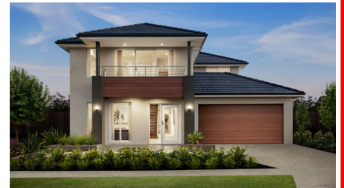
Front Façade Materials.
